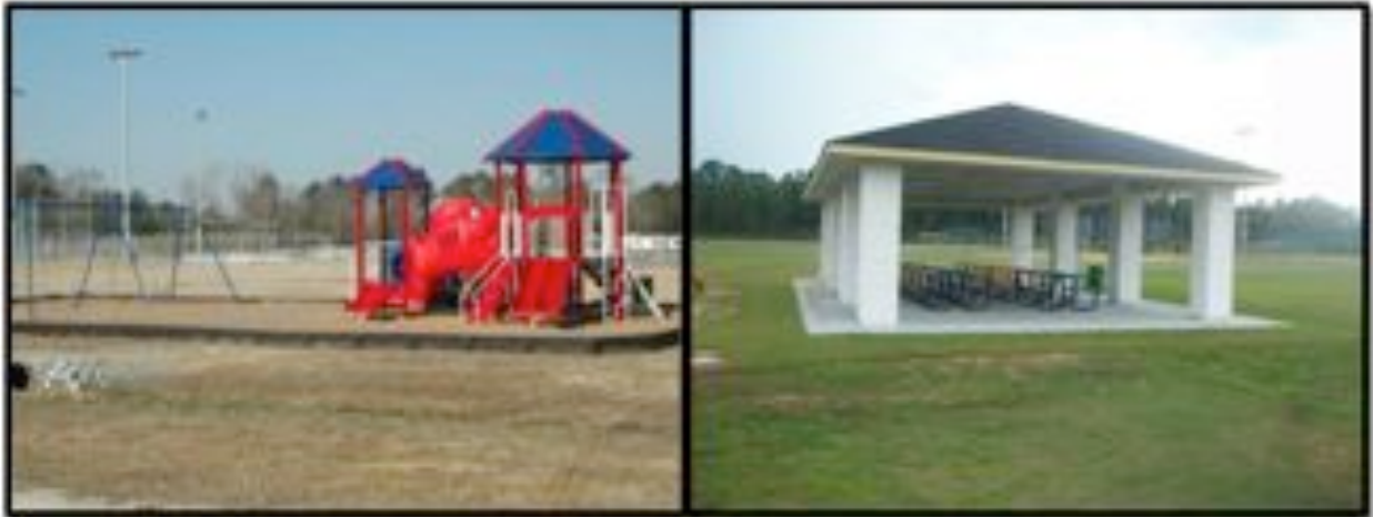
Figure 3. West Craven Park playground (left) and picnic shelter (right).
